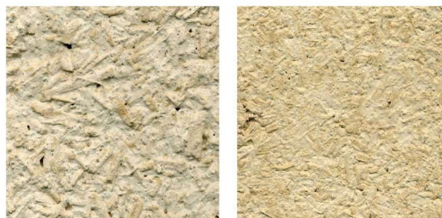
Fig. 6 : Two samples of lime plaster with different fibers size (Mazhoud et al., 2016)
