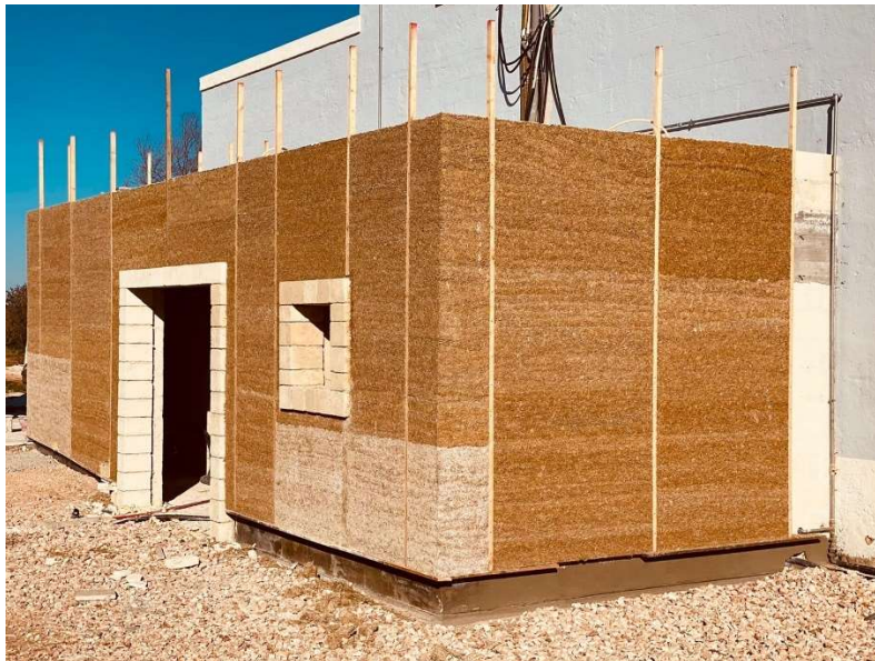
Fig.5 – Typical straw-bale house ( www.terrabuildingdesign.it )
