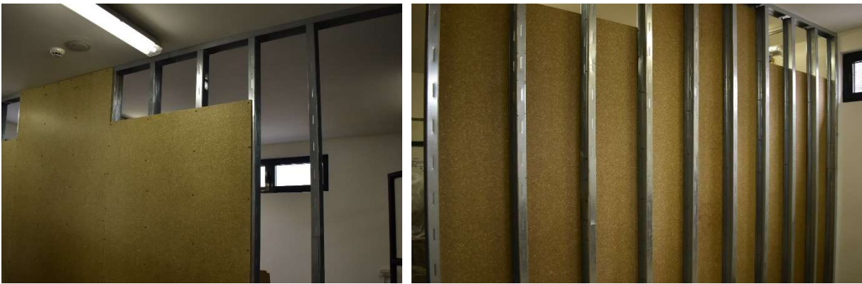
Fig.4 Wooden-steel panel framework (internal partition).
