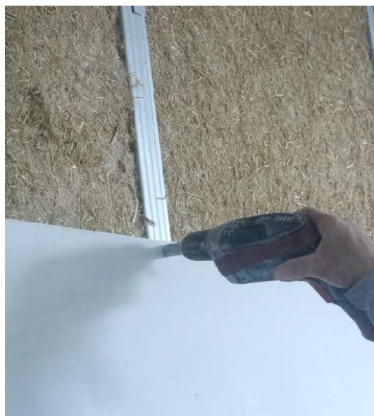
Fig.3 Details of the ricestraw panels.
