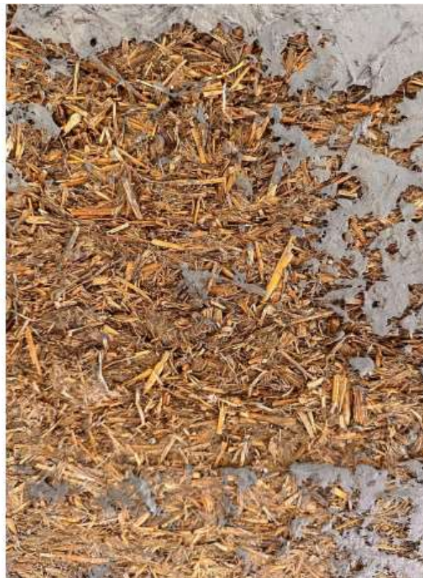
Fig.8 Finishing layer application by a mud plaster with straw aggregates.
