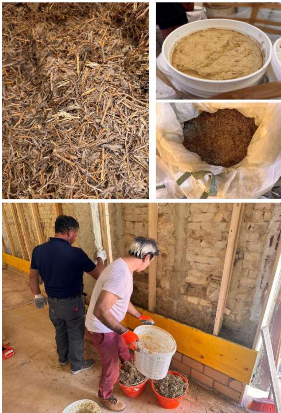
Fig.5 Lime straw mix filling.
