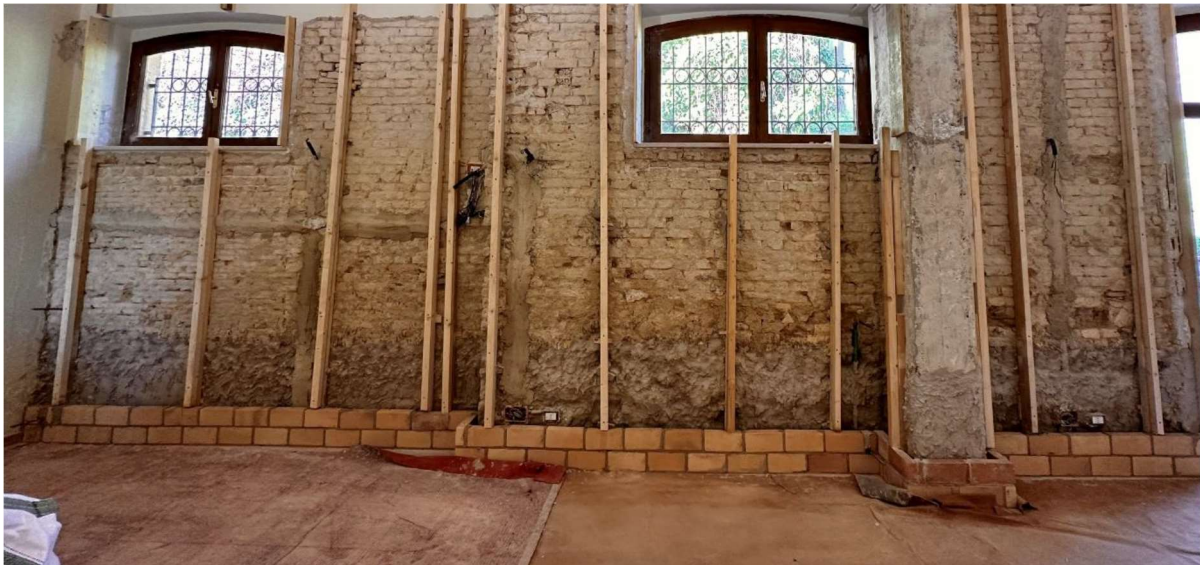
Fig.4 Fired bricks wall after preliminary phase: wooden framework application.
