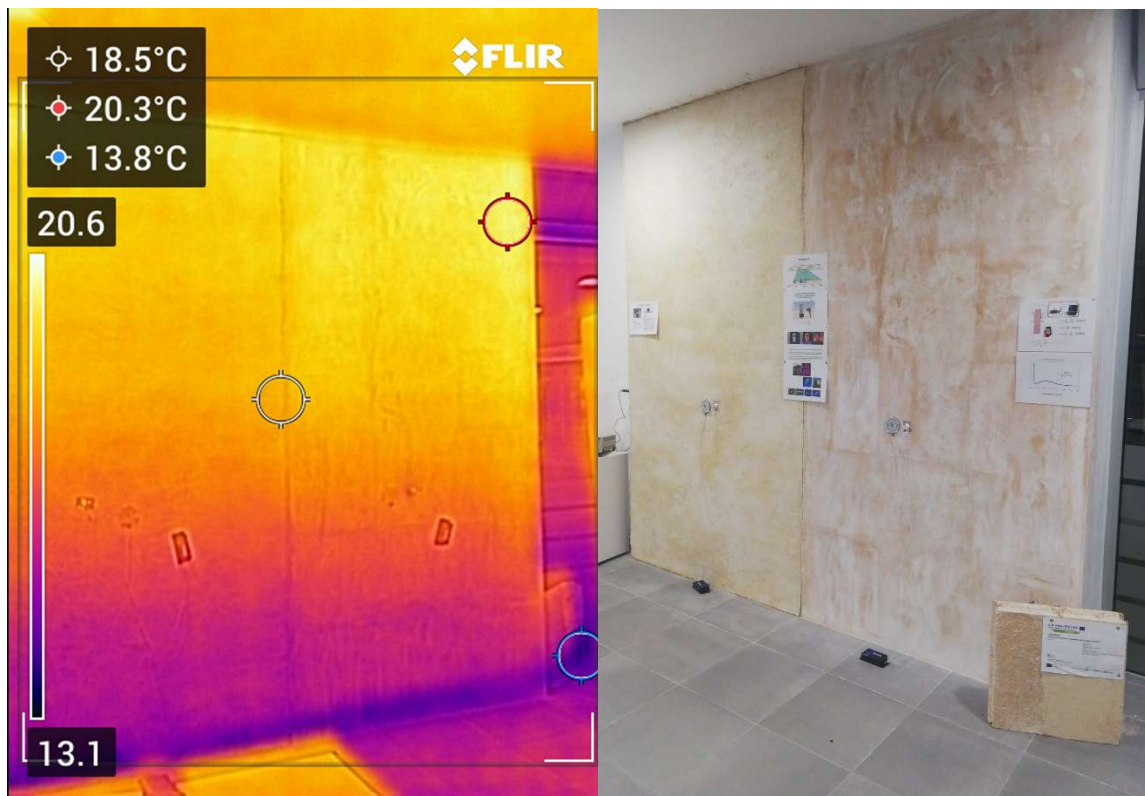
Fig. 6 Monitoring systems of the prototypes (from left to right: infrared thermal camera, thermal flux meter).
