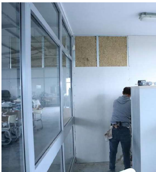
Fig.3 Details of the ricestraw panels.
