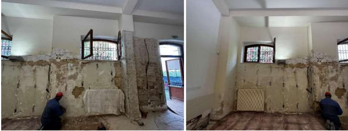
Fig.3 Preliminary phase: breaking existent plaster
