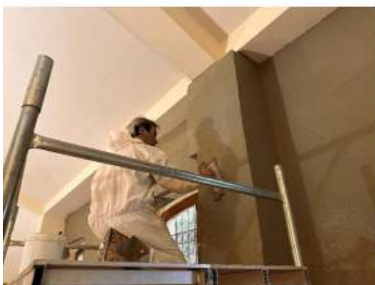
Fig.8 Finishing layer application by a mud plaster with straw aggregates.
